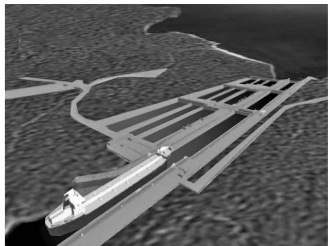
**Fig. 3.** Third locks design with water-saving basins and rolling gates [Reprinted with permission from Autoridad del Canal de Panamá (ACP) 2006]
