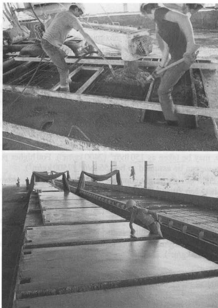
Casting and finishing precast concrete wall panels.
