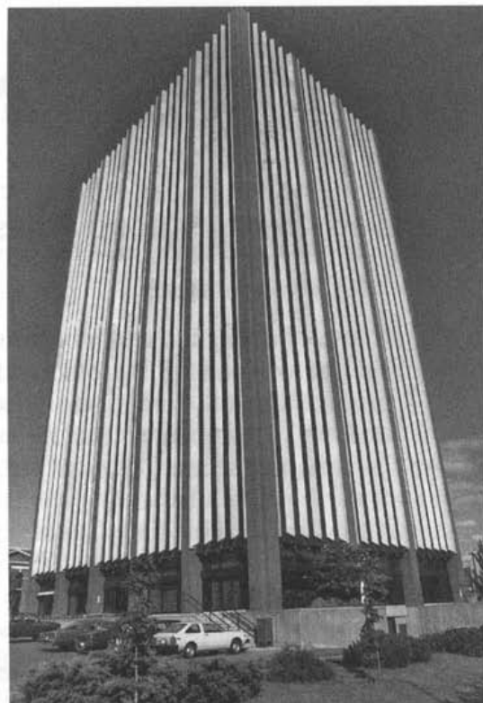
Reinforced concrete columns supporting an office building, Toronto, Canada.
