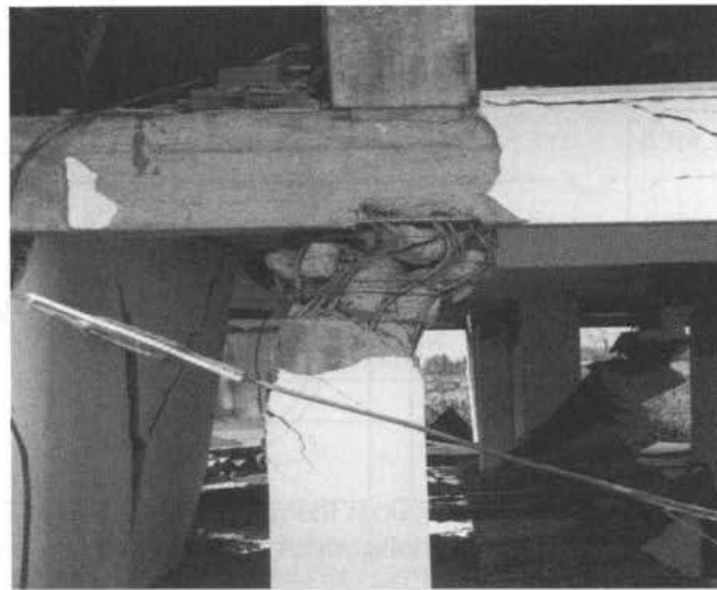
Lack of transverse reinforcement.
