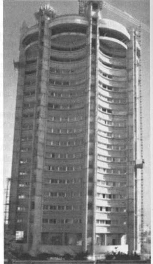
Curved beams in an office building.
