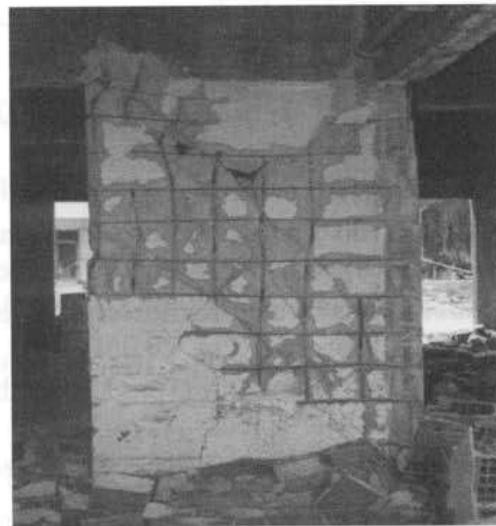
Shear wall after an earthquake.
