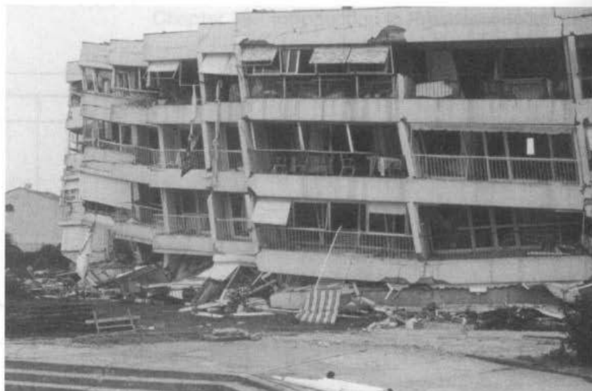
Collapse of frame concrete structures due to an earthquake.
