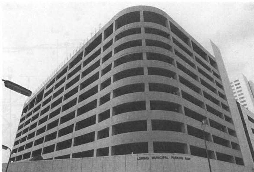
Reinforced concrete parking structure, Minneapolis, Minnesota.
