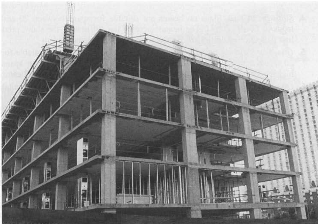
Flat-plate floor system.
