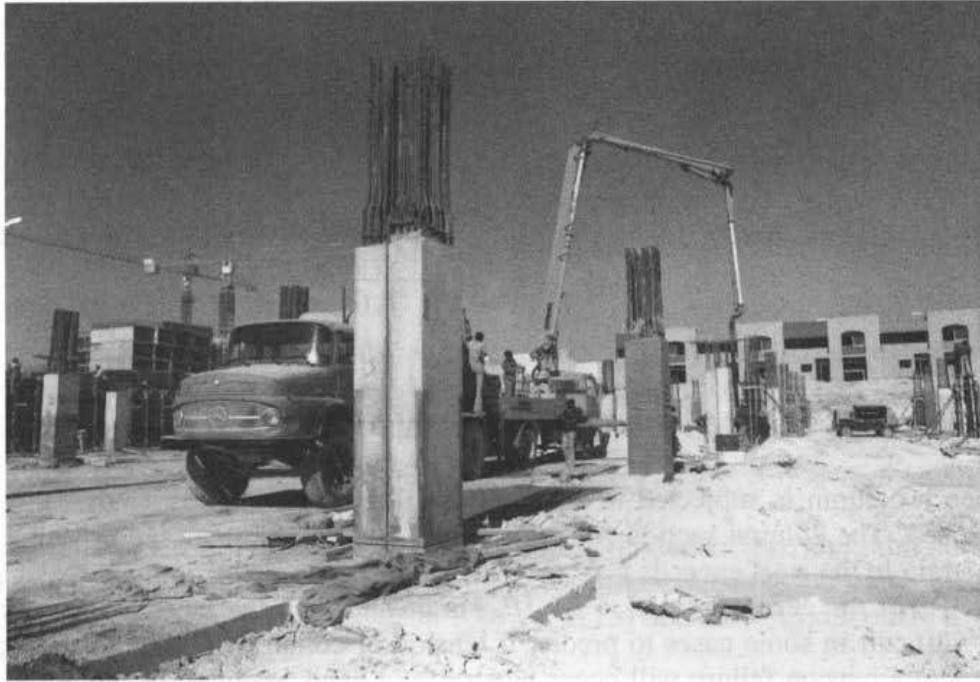
Reinforced concrete tied columns under construction. The two columns are separated by an expansion joint.
