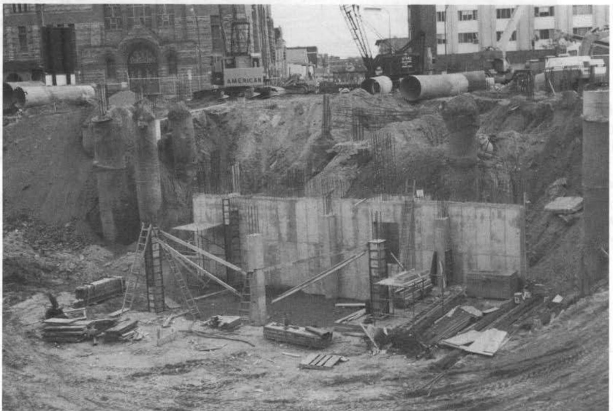
Wall and column footings, partly covered.
