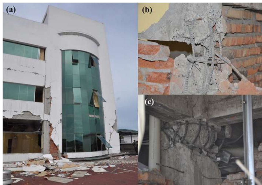
Fig. 14 a Damage to the building tower of the Solca hospital in Portoviejo, b failure of a non-structural column, and c shear failure of an interior column
