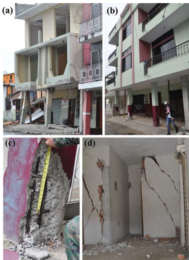
Fig. 7 Soft-storey buildings in Manta (a), damage to the columns (c) and partitions (d)
