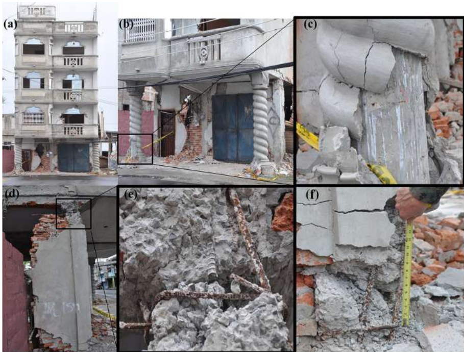
Fig. 8 4-storey RC building with several deficiencies located in Manta (a), structural irregularities and heavy cladding (b, c), and detailing deficiencies (d, e, f)
