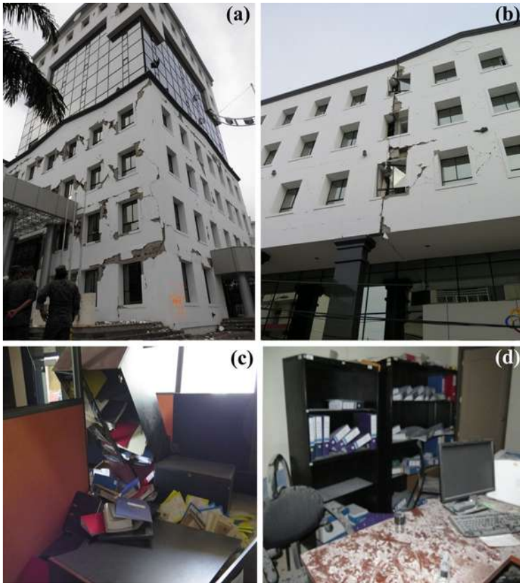
Fig. 12 a Exterior damage to the Supreme Court building, b pounding at the construction joint, c non-structural damage at upper stories and d at lower stories
