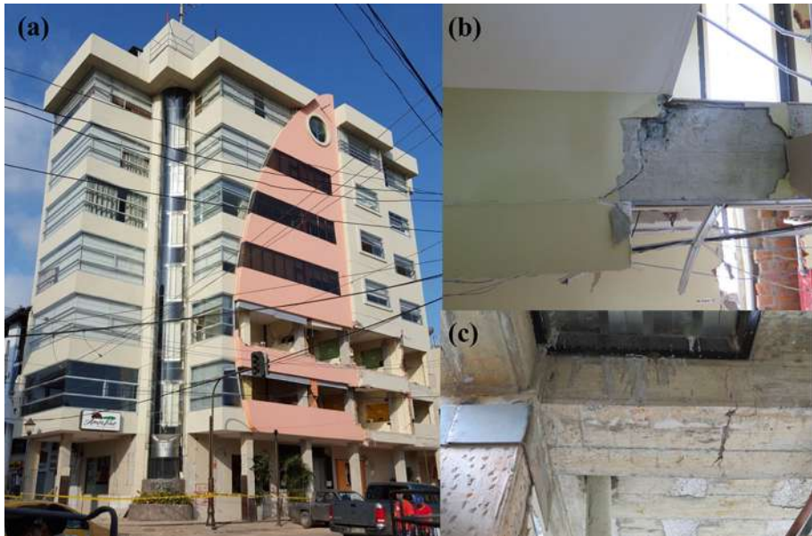
Fig. 10 7-storey Hotel Ceibo Dorado in Portoviejo overall damage (a), damage to the staircase (b) and perimetral beams (c)
