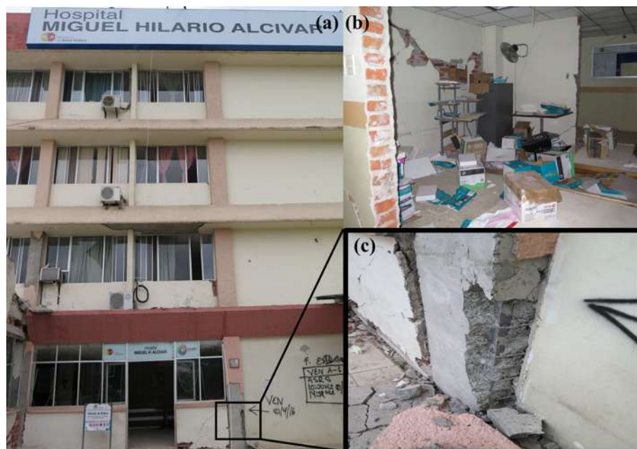
Fig. 13 a Damage to the retrofitted Miguel Hilario Alcivar hospital in Bahía de Caráquez, b interior damage to partitions and content, and c structural damage in the wall boundary
