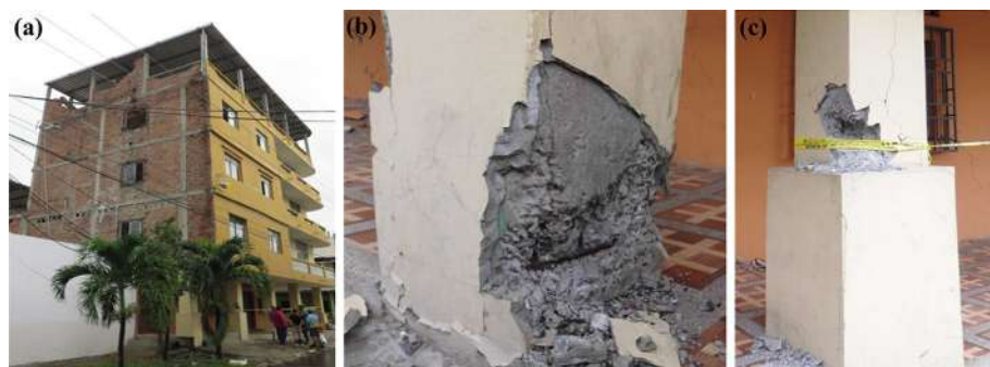
Fig. 6 5-Storey RC building with masonry infills located in Tarqui (Manta) (a), and its damage to the ground-floor-columns (b, c)
