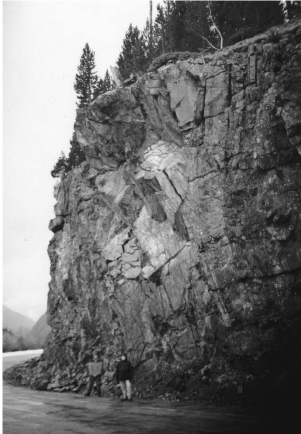
Fig. 1.4. Strata close to present a toppling failure mechanism, Benasque Valley, Huesca (Spain).
