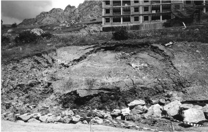
Fig. 1.5. Rotation slide in a slope close to Formigal, Huesca (Spain).
