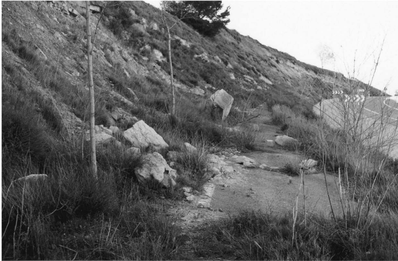
Fig. 1.3. Rockfalls in a slope close to Cenicero village, La Rioja (Spain).
